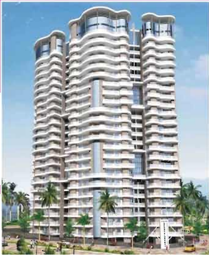
INLAND WINDSORS Airport Road, Maryhill, Mangalore 2 BHK: 1360 Sq.Ft. 3 BHK: 1755, 1825, 1950 Sq.Ft. Duplex: 2720, 2730 Sq.Ft.
